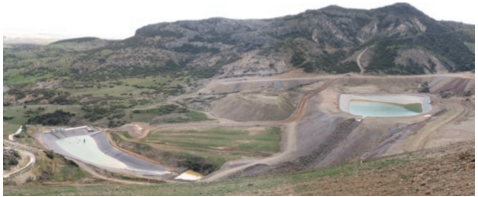
View of Kisladag Development Rock Pile and Runoff Collection Ponds, Looking South
