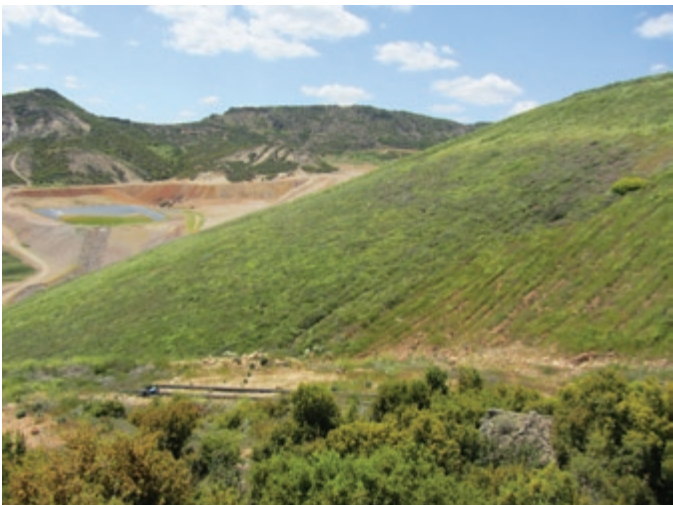
Top: View of Kisladag Development Rock Pile Looking North Bottom: Reclaimed Portion of Development Rock Pile on the West Portion of the Facility
