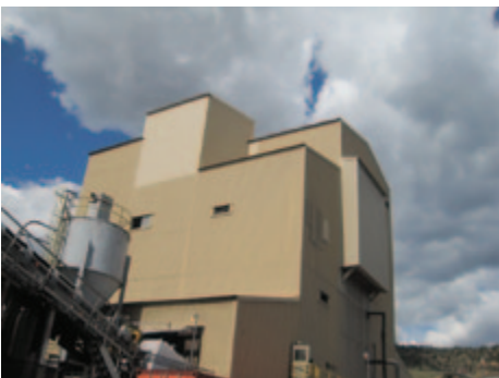
Existing New Elk Coal Company wash plant exterior
