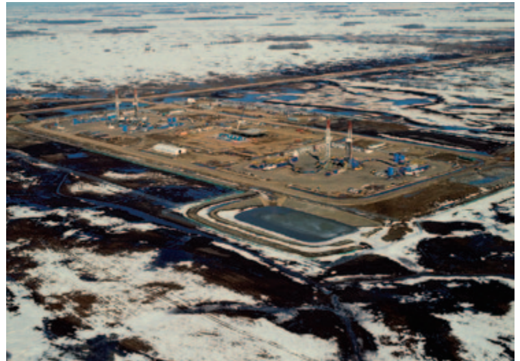
Aerial photograph of the BHP Billiton Jansen Project
