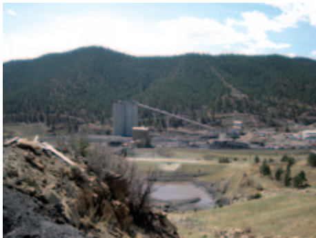
New Elk Coal Company surface facilities looking South
